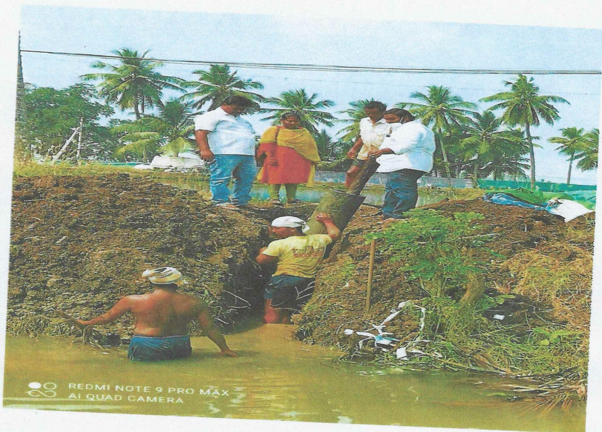
Remove outlet pipes in Thundurru Village of Bhimavaram Mandal from Thundurru Branch Channel
